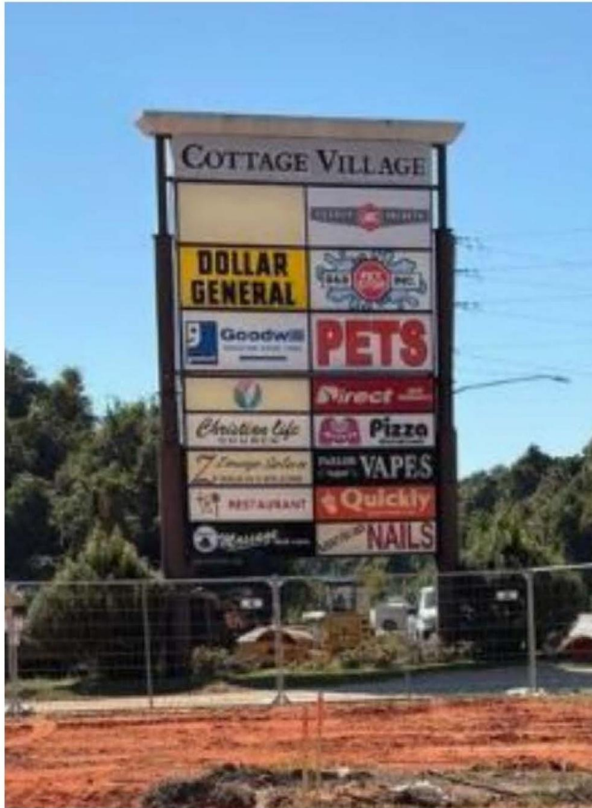
Existing Pylon Conditions
