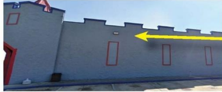
Former north wall
