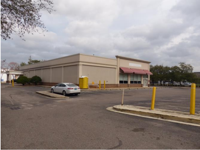
1. View northeast to the west (left) and south (right) elevations of the existing drug store building on the property
