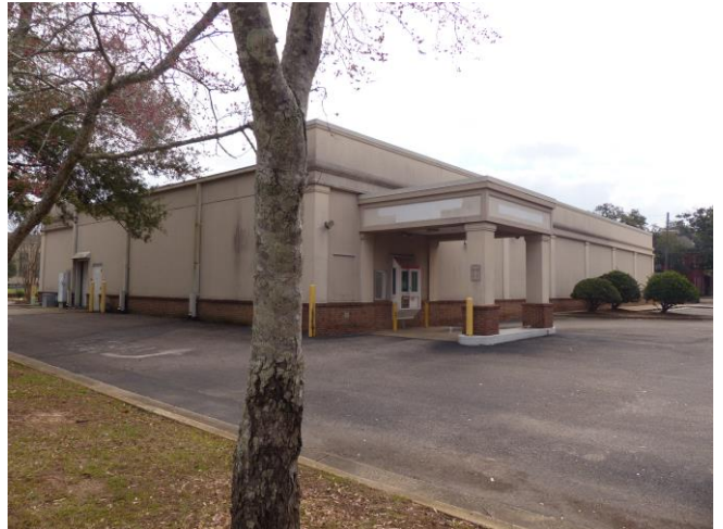
4. View southeast to the north (left) and west (right) elevations of the existing building
