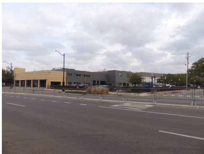
17. View northeast across Broad Street from the northeast corner of the property
