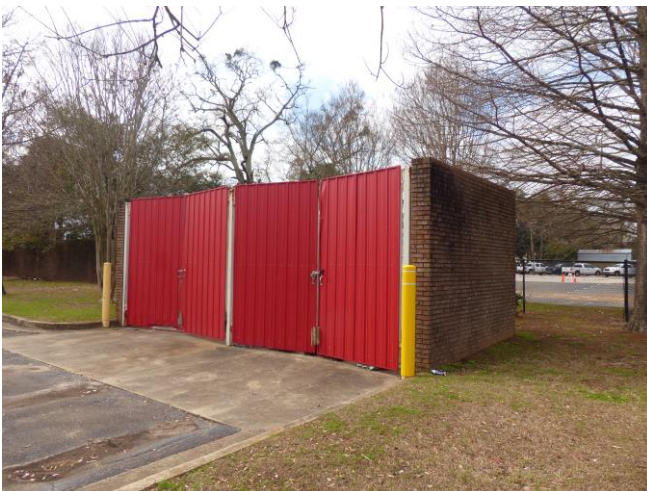
5. View southwest to the existing dumpster enclosure at the northwest corner of the property
