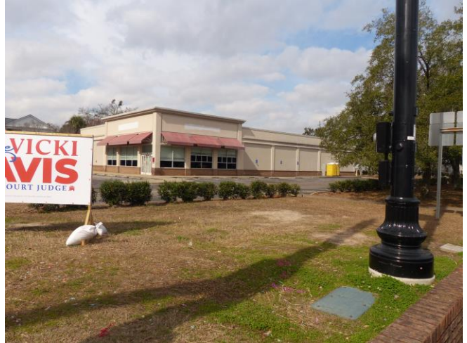
2. View northwest to the south (left) and east (right) elevations of the existing building on the property
