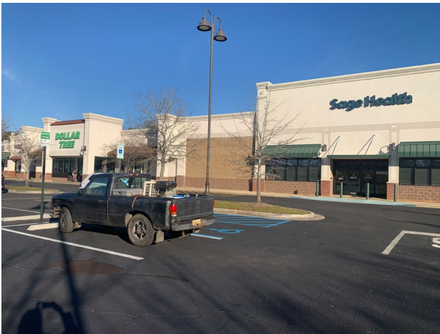
3. View of shopping center, looking northwest.
