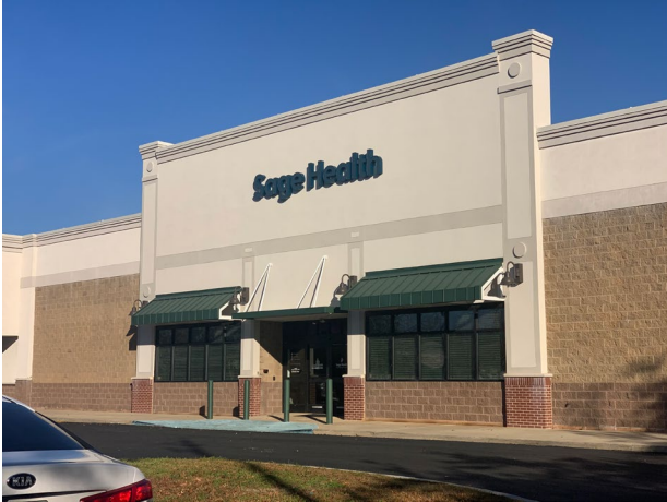
1. View of façade, looking northwest.
