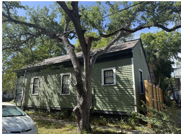
6. South elevation of property with section of E fence, looking N.
