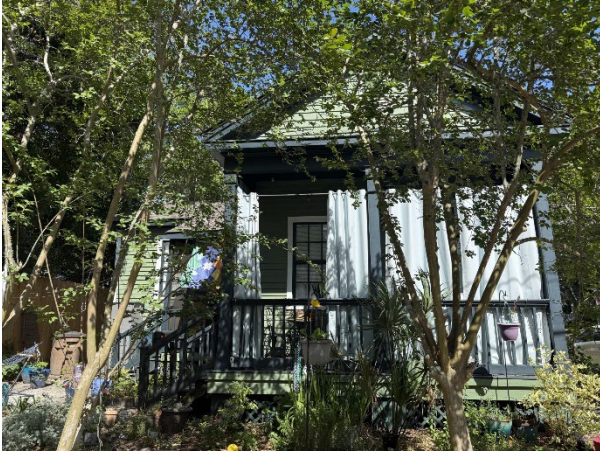
1. West façade of subject property, looking E.
