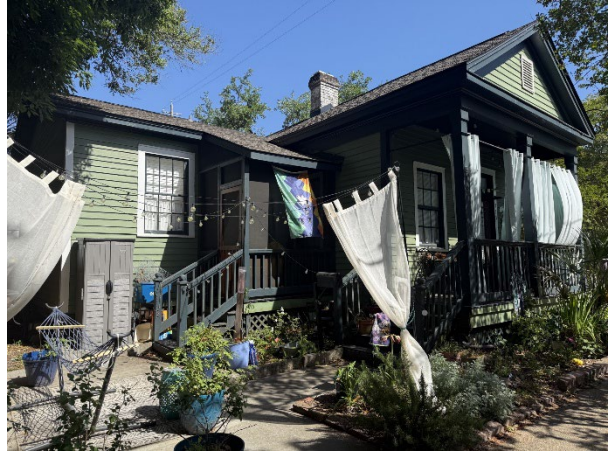
2. NW view of property looking SE.
