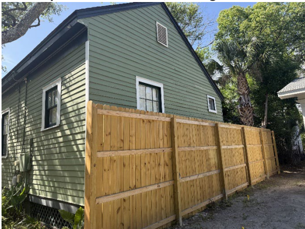
5. View of fence on E property line, looking N.
