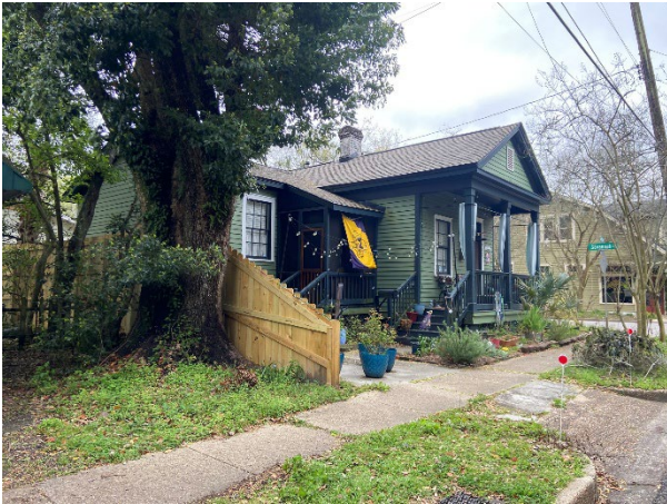
3. View of tapered fence behind front plane of residence, looking SE.
