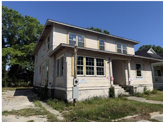
4. View of west and north elevations, looking SE.
