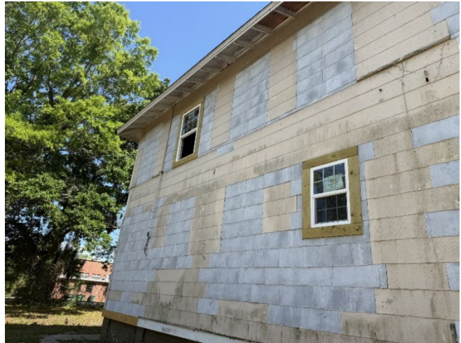
8. View of deleted windows on the north elevation.
