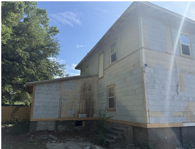
9. View of east/rear elevation of the property, looking SW,
