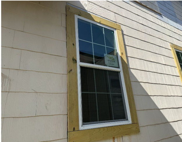
7. View of vinyl window and trim on the north elevation.
