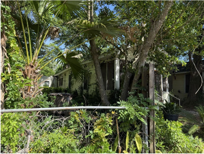
3. View of north elevation, looking SE
