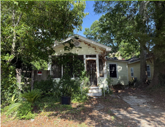
1. View of west façade of property, looking E
