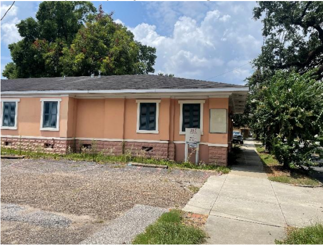
3. East elevation, looking W
