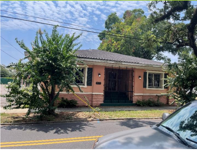
1. North (primary) façade, looking S
