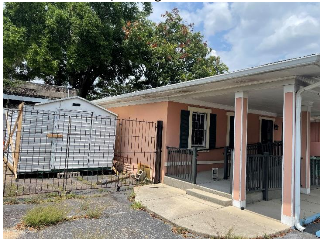
6. South (rear) elevation and metal accessory structure in rear yard, looking NW
