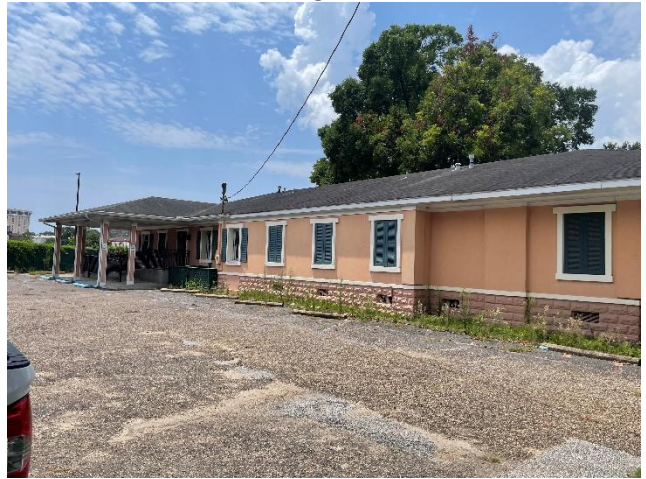
4. East elevation, looking SW
