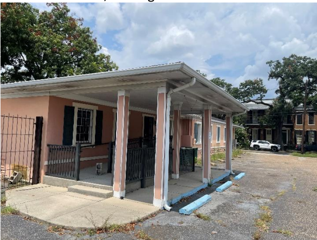
5. East elevation, looking NW
