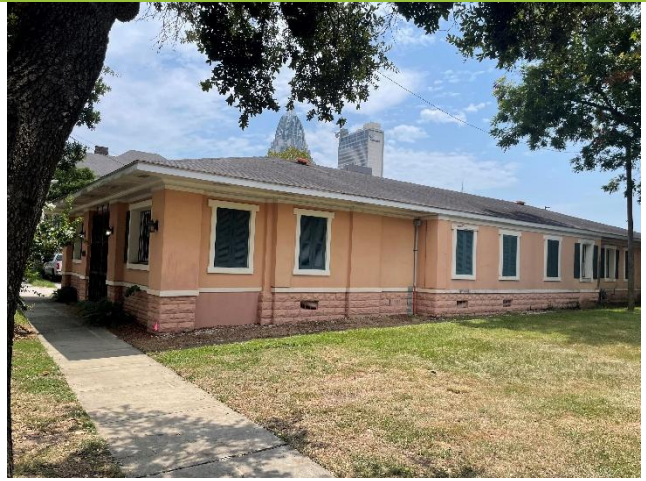
2. West elevation, looking SE
