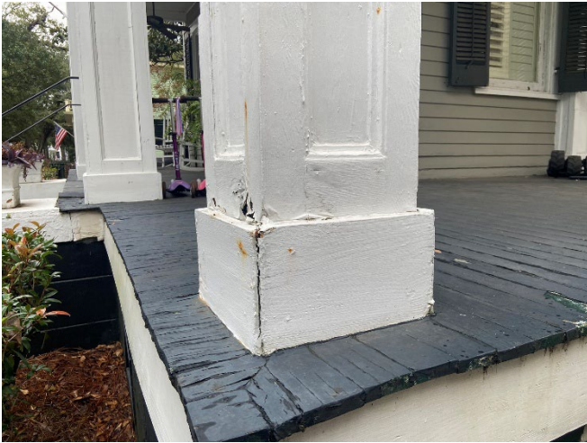
9. Column S1, wood rot at previous dutchman repair
