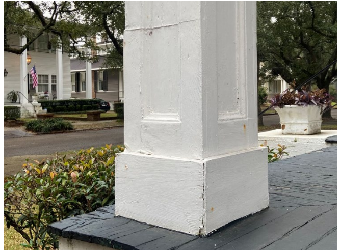
10. Column S1, wood rot at previous dutchman repair
