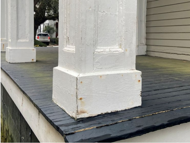
13. Column S4, wood rot at replacement base
