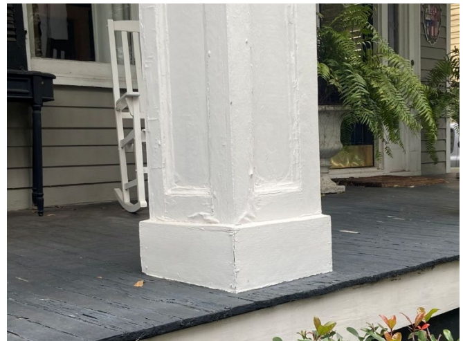
6. Column E2, bubbling paint at base of shaft
