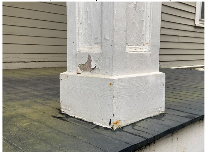
12. Column S3, wood rot at base and paint failure at bottom of shaft
