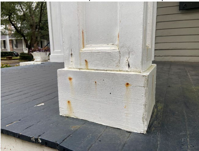
11. Column S2, wood rot at bottom of shaft
