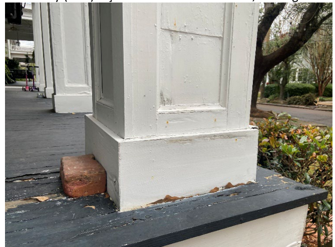
4. Column E1, wood rot at previous dutchman repair
