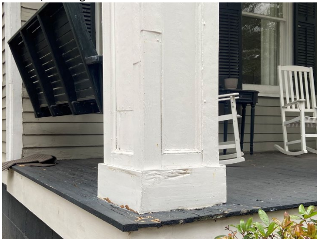
5. Column E1, rot at replacement base
