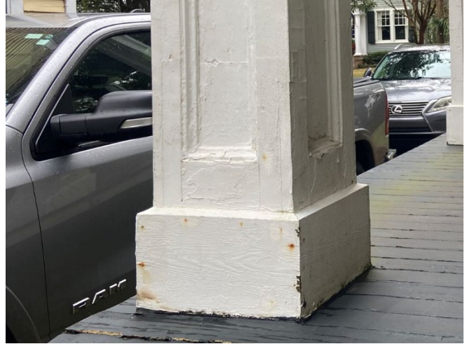
14. Column S4, wood rot at replacement base
