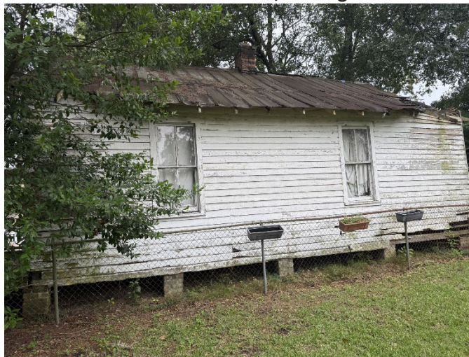
4. View of north elevation, looking S
