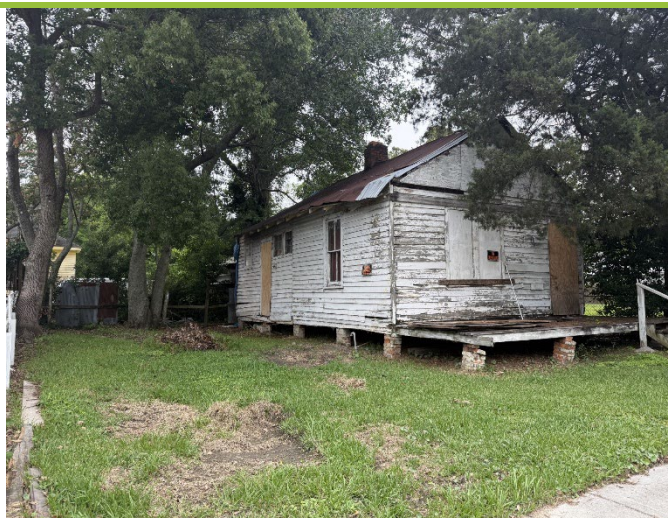
2. View of property, looking NW
