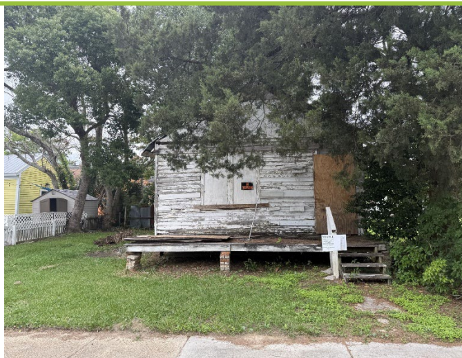
1. View of east façade of property, looking W
