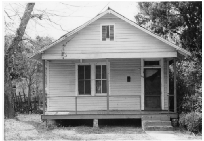
9. East façade of property from 1989 survey photo.
