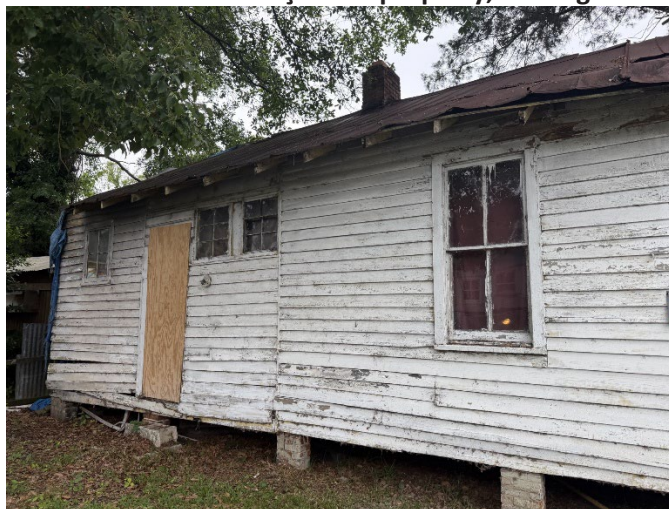
3. View of south elevation, looking NW
