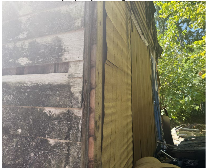
4. View of northwest corner of structure (rear), looking S
