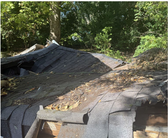
5. View of rear of property
