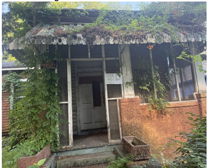
6. Detail of façade, looking W
