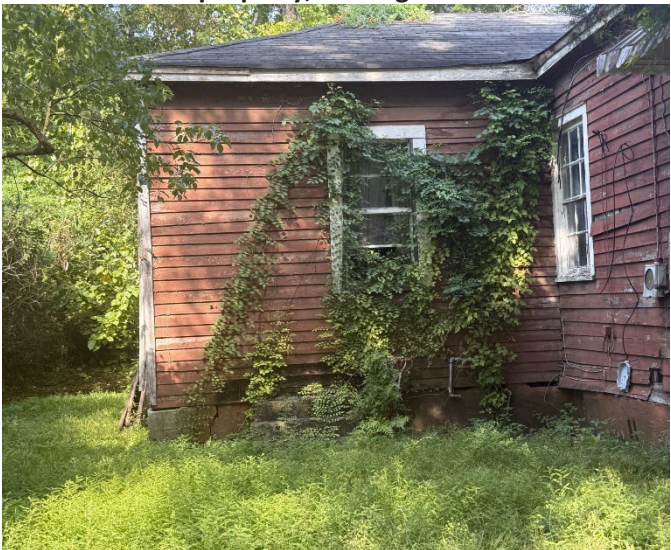
3. View of south elevation, looking NW
