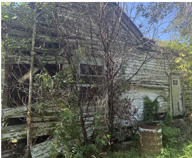
5. View of rear (north) elevation, looking SW
