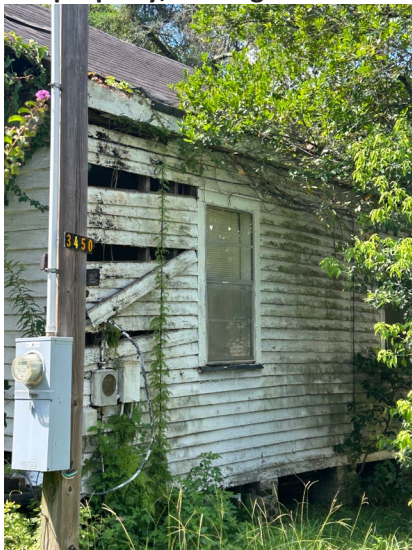
3. View of east elevation, looking NW
