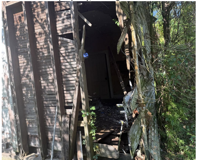
4. View of rear (north) corner of east elevation, looking W
