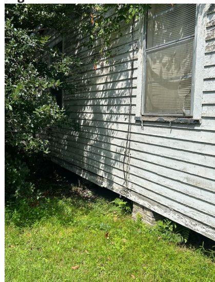
6. View of west elevation, looking NE
