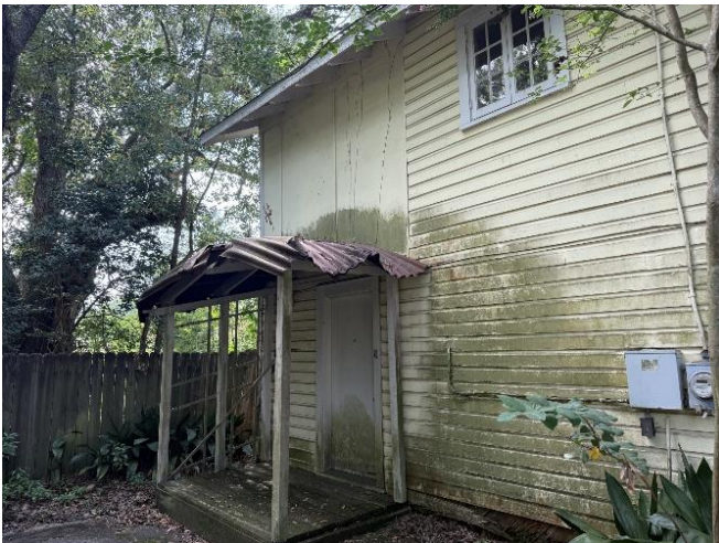
5. Rear entrance to garage apartment on north elevation, looking southeast
