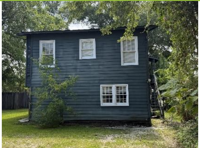
2. West façade of accessory building, looking east. Garage doors have been infilled.
