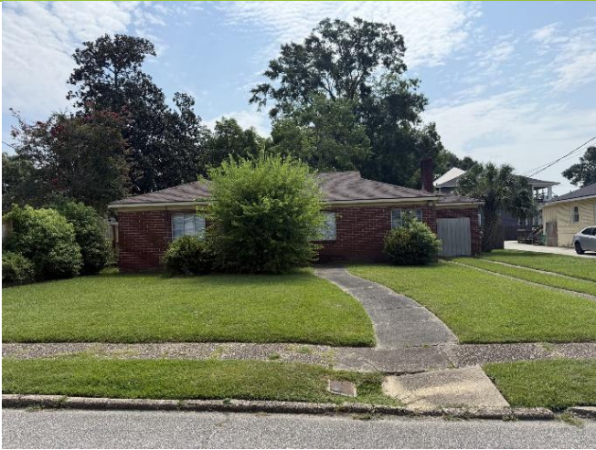
1. West façade, looking east.
