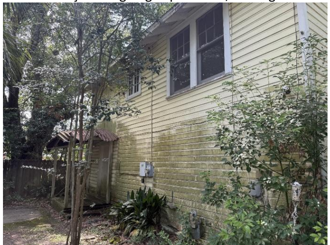
4. North elevation of garage apartment, looking southeast
