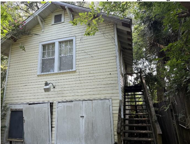
3. South entrance stair, looking east
