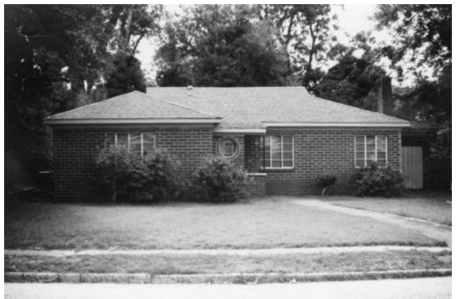
6. Survey photograph of west façade, looking east, June 1984.
