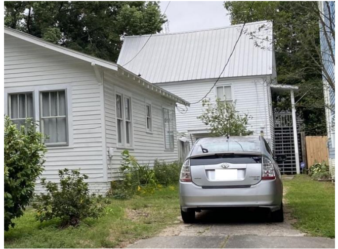
8. Garage apartment at 52 Le Moyne Place, looking east.
