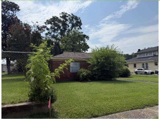
2. West façade, looking southeast. 69 Bradford Avenue in background.
