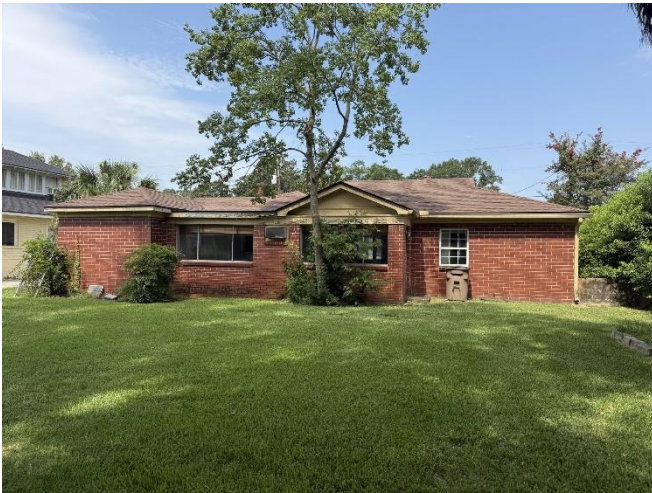
3. East (rear) elevation, looking west.
