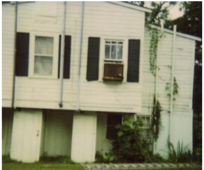
6. North elevation of accessory building, looking south, date unknown (c. 1994)
