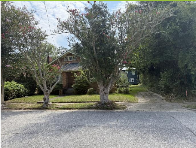
1. West façade of primary dwelling, looking east
