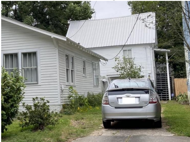
9. Garage apartment at 52 Le Moyne Place, looking east.
