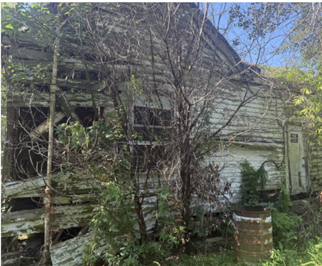
5. View of rear (north) elevation, looking SW
