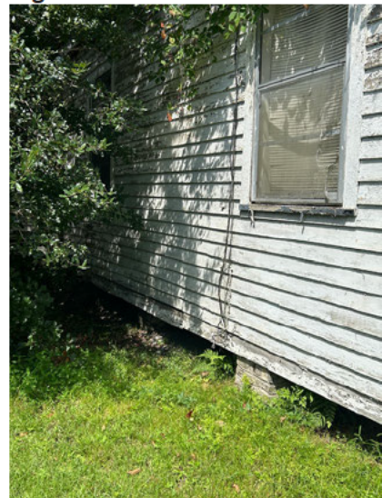
6. View of west elevation, looking NE
