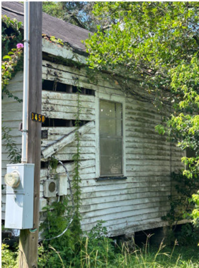
3. View of east elevation, looking NW
