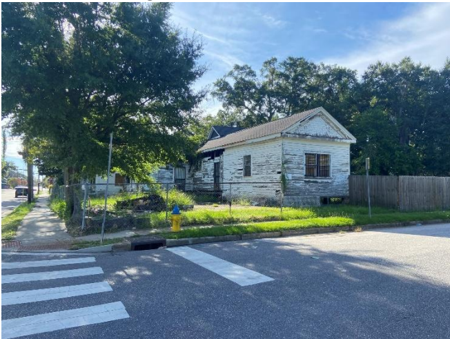
3. North and west elevations of c. 1905 shotgun facing Marine Street, looking SE
