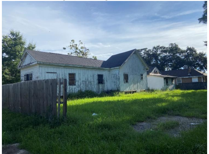
4. South (rear) elevation of c. 1905 shotgun (left) and c. 1942 addition (right), looking NE
