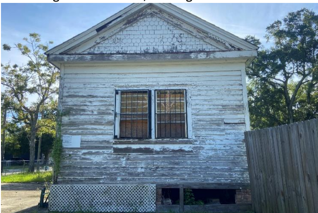
5. West gable end of c. 1905 shotgun, showing surviving fish scale shingles
