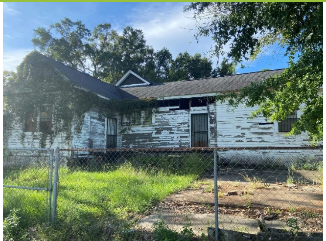
2. North façade of c. 1905 shotgun (left) and c. 1942 additions (right), looking S
