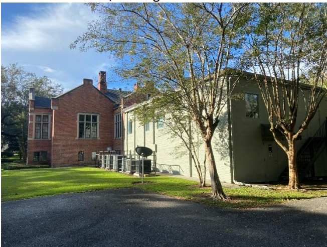
5. Rear addition (right) and north elevation (left), looking S
