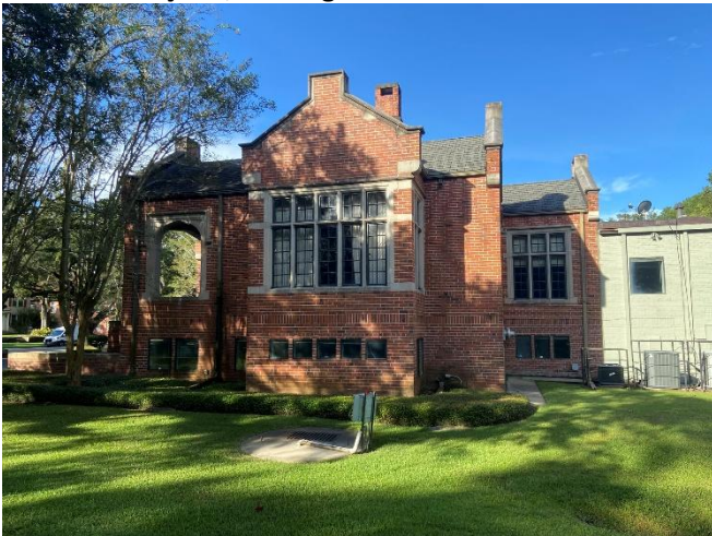
3. East elevation, looking W
