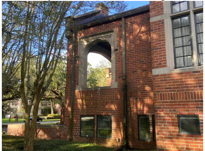
4. Arched opening at east end of front porch
