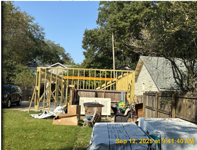
3. View of property, looking W
