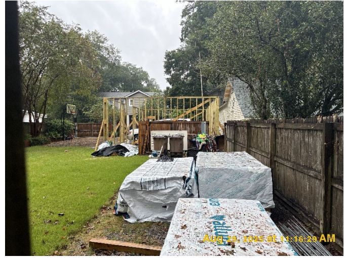
2. View of property, looking W
