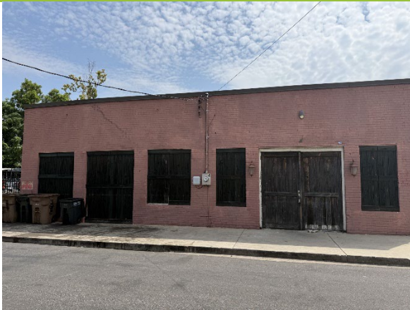
1. West façade of 4 N Cedar Street, looking E.
