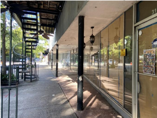
3. 310 Dauphin, existing recessed storefront, looking W
