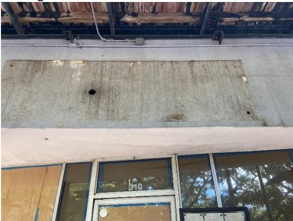
5. 310 Dauphin, existing stucco façade wall
