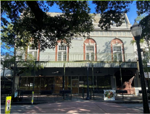
1. South façade of 310 Dauphin, looking N
