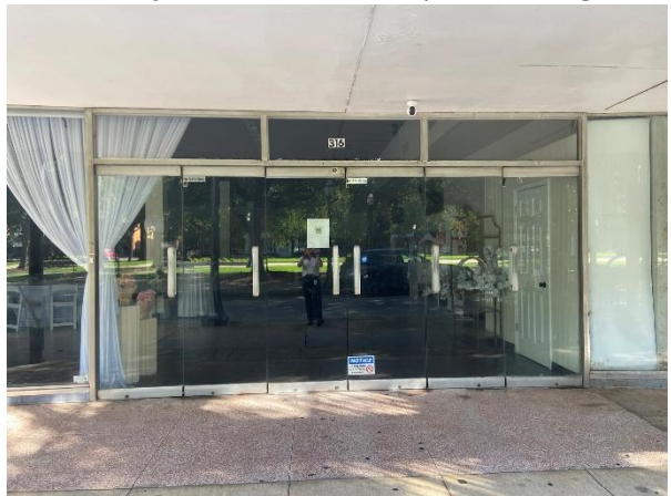
10. 316-318 Dauphin, possible original (c. 1960) doors
