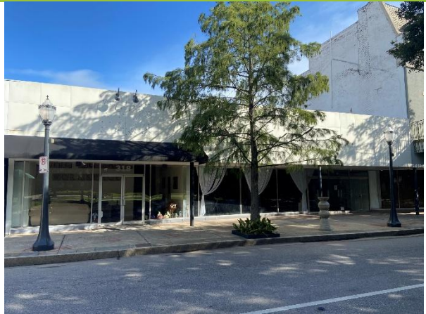
8. South façade of 316-318 Dauphin, looking N
