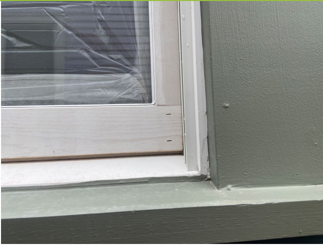
13. Detail of replacement one-over-one windows.
