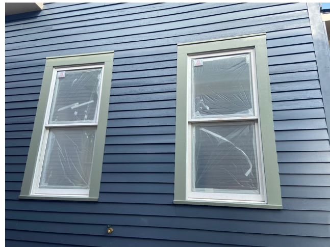
12. Detail of replacement one-over-one windows.
