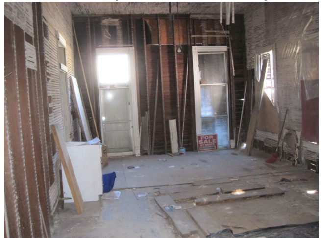
6. Interior view of box head windows in place (May 2024)
