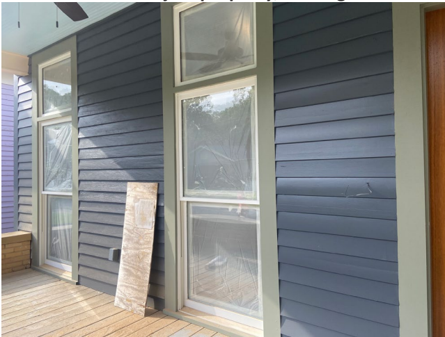
3. Detail of replacement windows on façade
