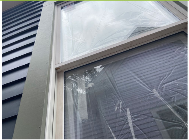
14. Detail of replacement one-over-one windows.
