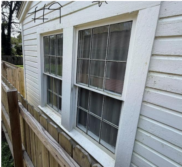
17. Windows #9 & 10, north elevation
