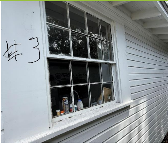
13. Window #3, south elevation
