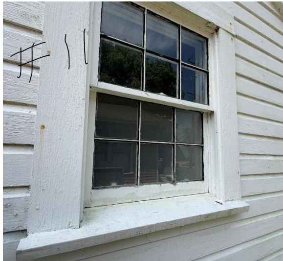
18. Window #11, north elevation
