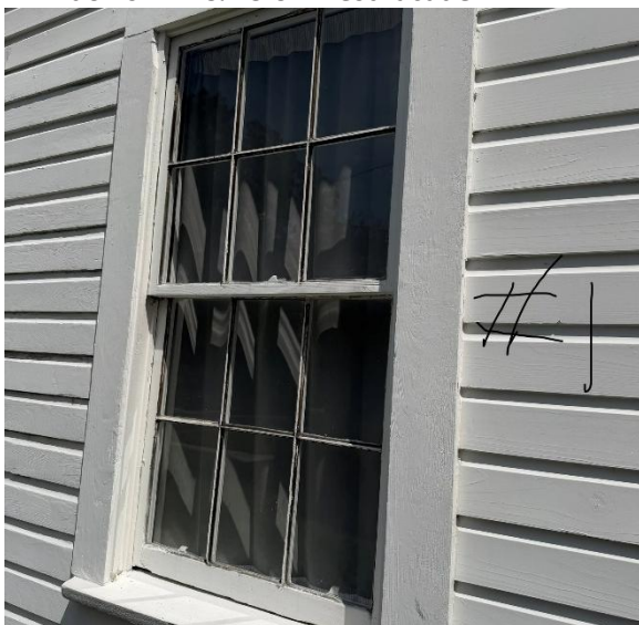
11. Window #1, south elevation
