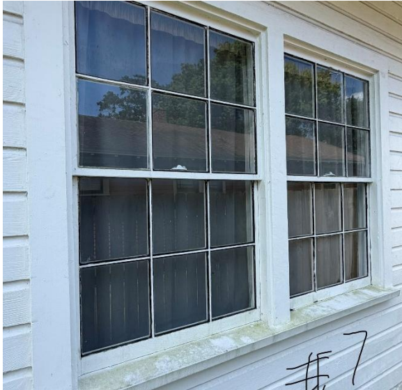
15. Windows #6 & 7, north elevation
