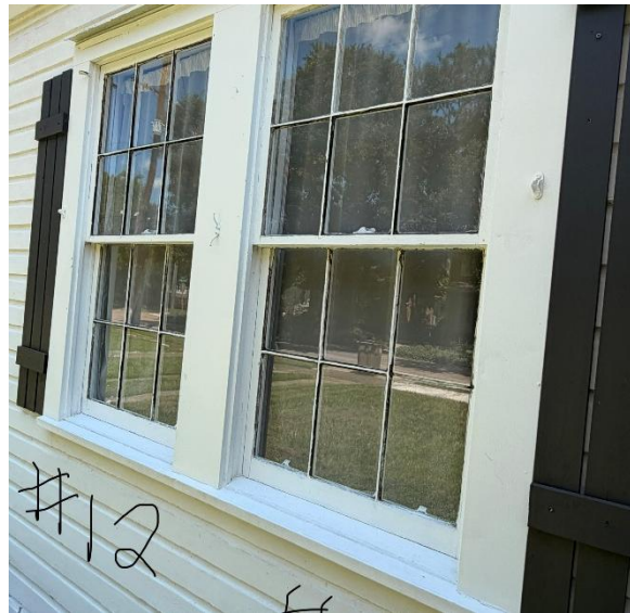
10. Windows #12 & 13 on west facade
