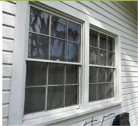
14. Windows #4 & 5, east (rear) elevation
