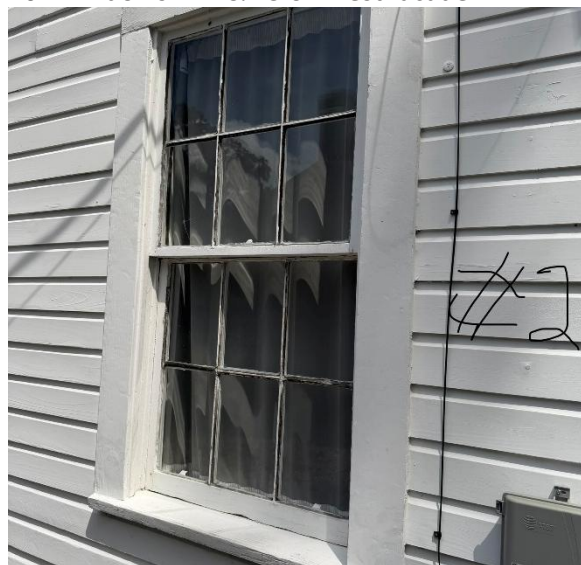
12. Window #2, south elevation
