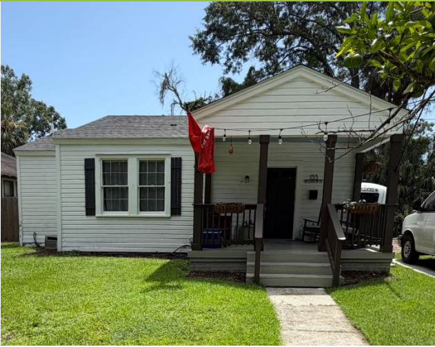
1. West façade, looking SE
