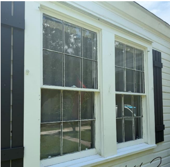
9. Windows #12 & 13 on west facade
