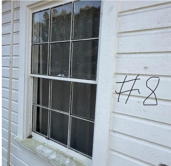
16. Window #8, north elevation
