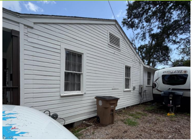
2. South elevation, looking NE
