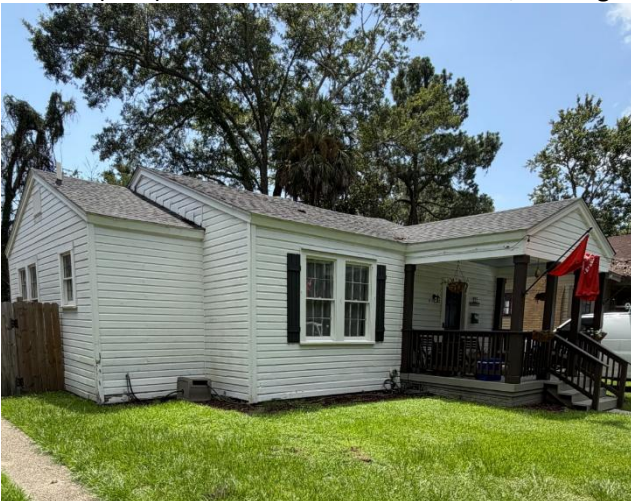
5. West façade and north elevation, looking SE
