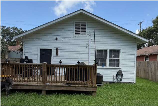
3. East (rear) elevation of c. 1960 addition, looking W
