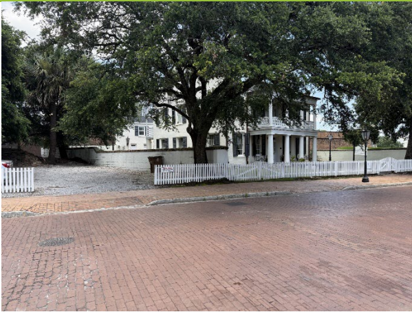
7. 104 Theatre Street and masonry wall, looking N.
