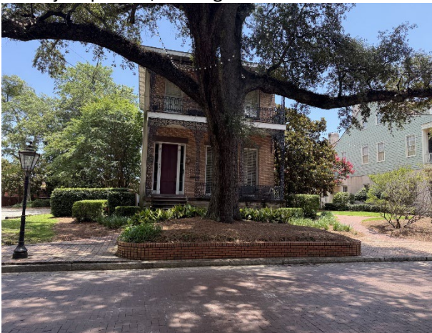
5. East façade of 163 St Emanuel Street
