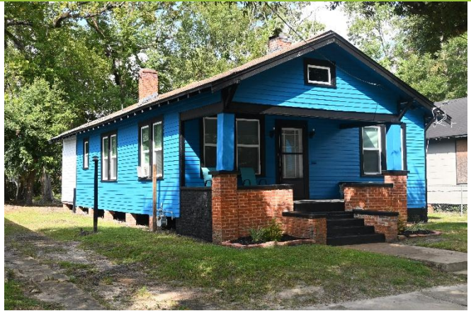
2. South façade and west elevation, looking NE
