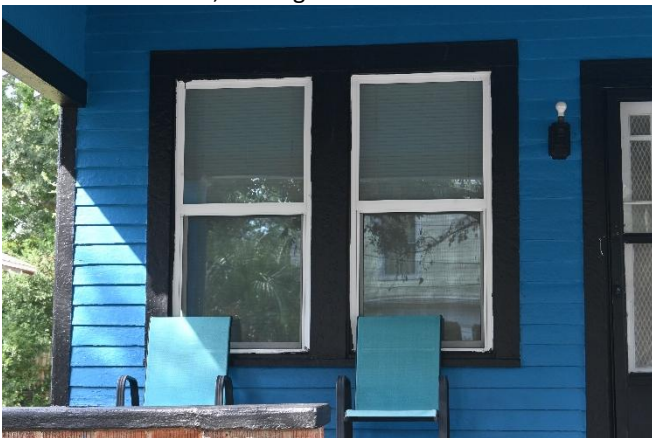
5. Closeup of vinyl replacement windows on south façade at front porch. Windows appear to fit the existing opening.
