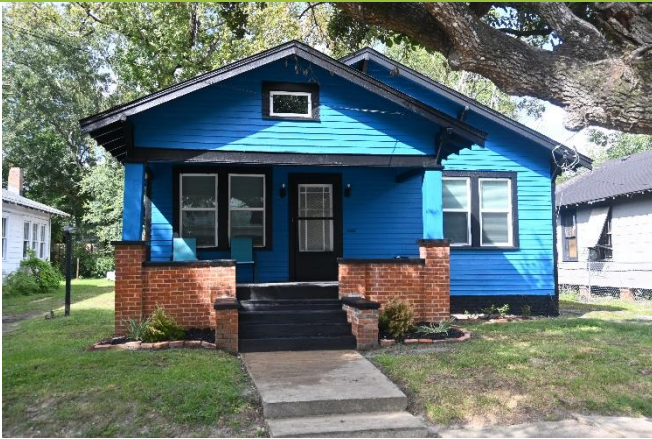
1. South façade, looking N
