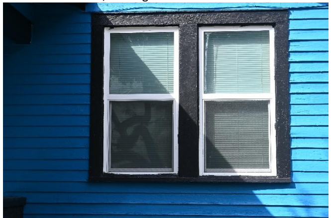
6. Closeup of vinyl replacement windows on south façade. Windows appear to fit the existing opening.
