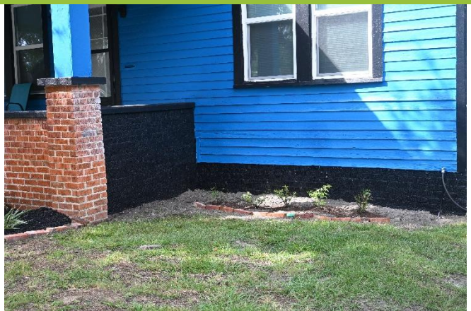
8. East knee wall of porch and foundation painted black.
