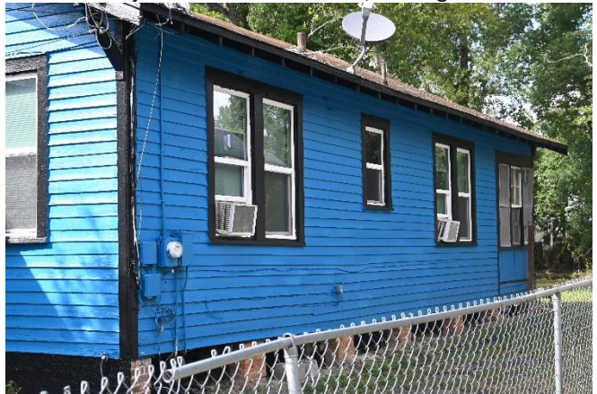
4. East elevation, looking NW
