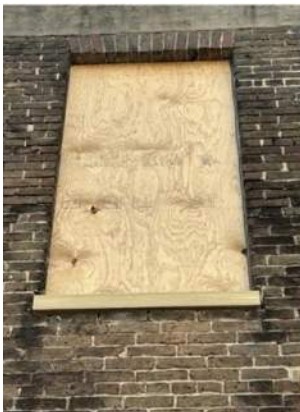
9. Representative window 2L Second floor, north elevation
