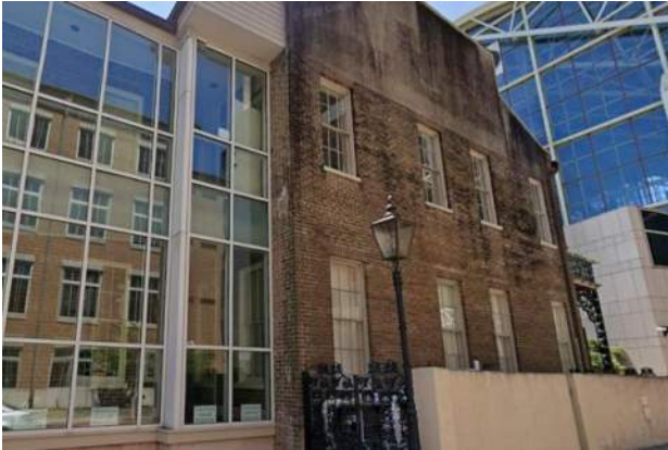
3. North elevation, looking SW
