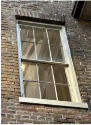
7. Representative window 2B Second floor, south elevation
