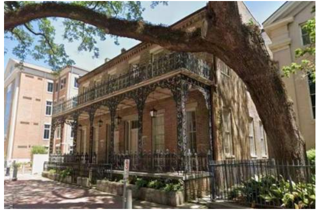
2. West façade and south elevation, looking NE
