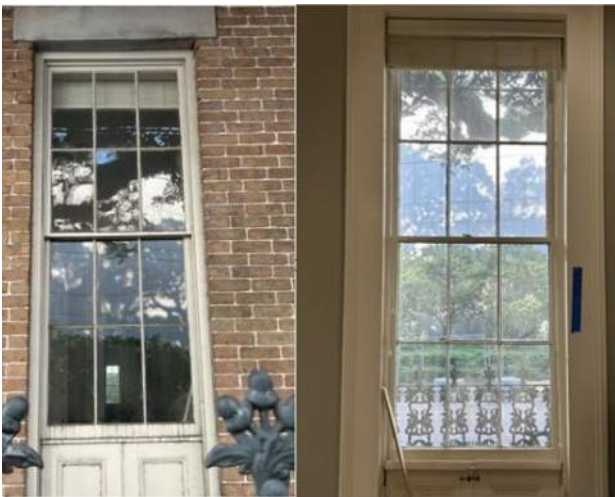
5. Representative window 1F First floor, west façade
