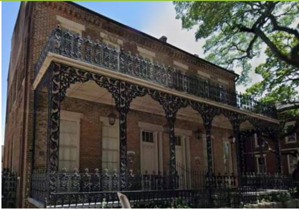
1. West façade, looking SE
