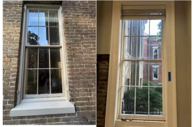
4. Representative window 1B First floor, south elevation
