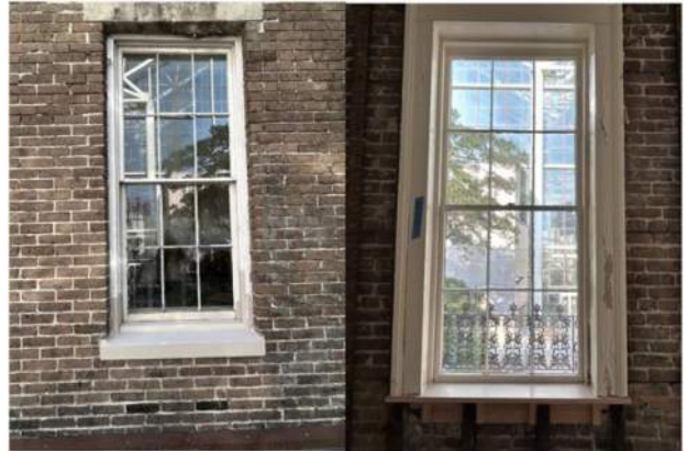
8. Representative window 2I Second floor, west façade
