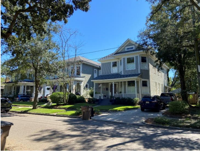
7. 1207 Selma Street, looking S
