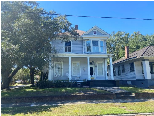
5. 308 Rapier Avenue, looking W
