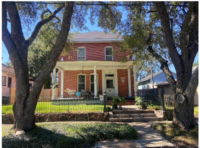
6. 304 Rapier Avenue, looking W
