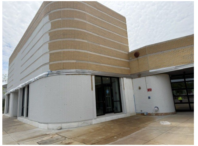
4. View of north and west elevations, looking E (taken on April 22, 2026)
