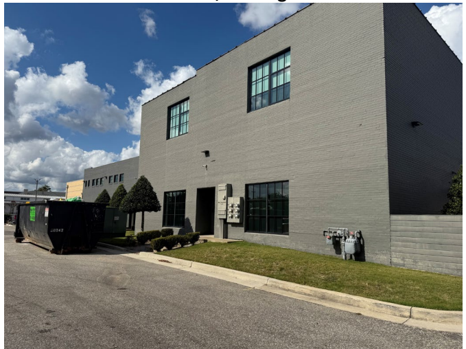
10. View of south elevation, looking NW
