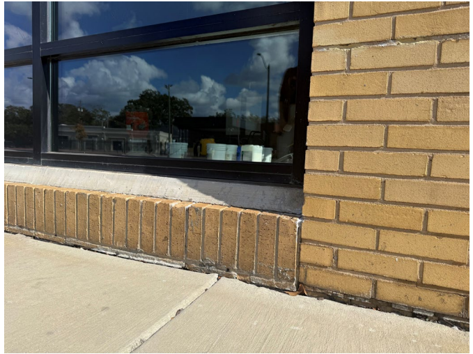
14. Detail on contrasting brick on west elevation
