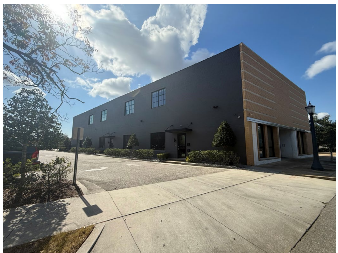
12. View of north and east elevations, looking SW
