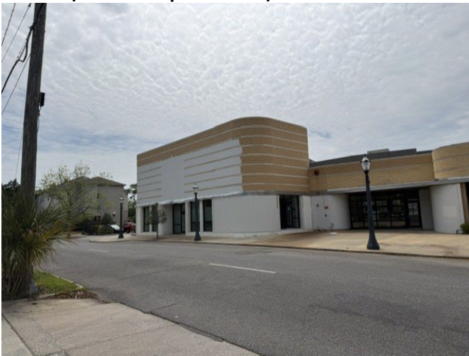
3. View of north elevation, looking SE (taken on April 22, 2026)
