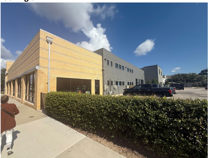
11. View of south and west elevations, looking NE
