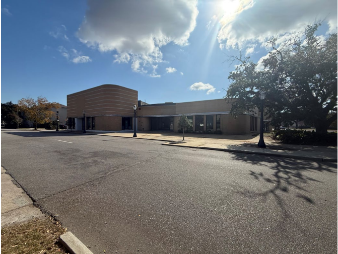
7. View of property's north façade, looking SE
