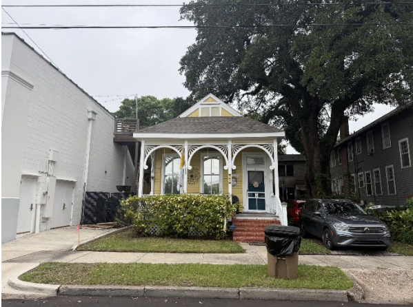
1. West façade, looking E.
