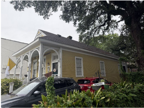
4. South elevation of existing structure, facing N.
