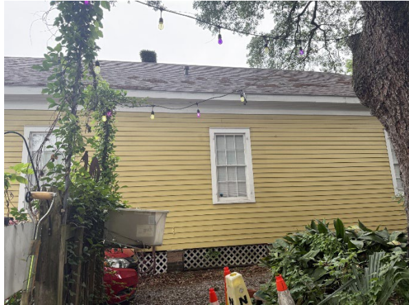
5. Location of proposed south addition, looking N.
