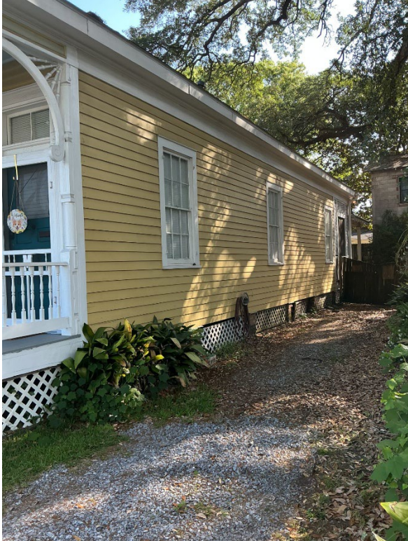
8. View of south elevation, looking W.
