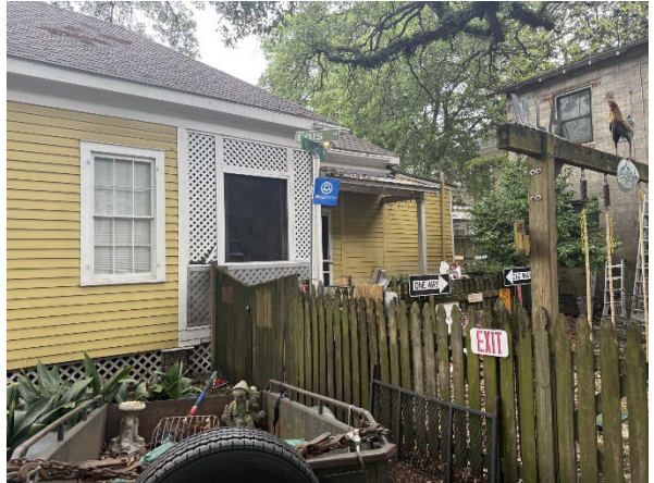
6. Location of proposed east addition, looking NE.
