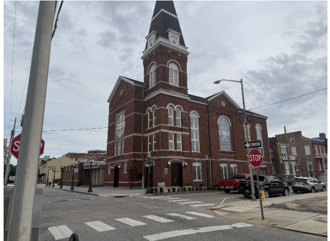
5. View of 251 St Francis, directly south of subject site.
