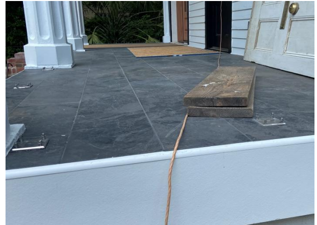
10. New tiles on south porch deck
