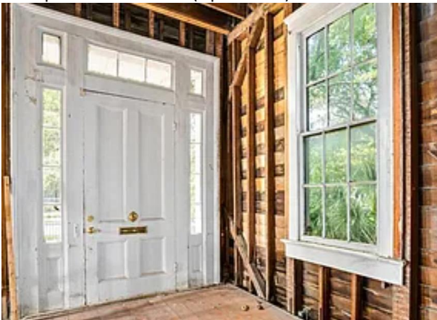
5. Interior of historic entry door (2020)
