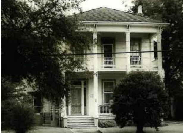
1. Primary (south) façade, looking north (1983)
