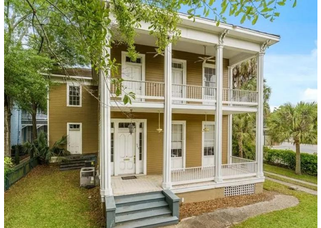
2. South façade, looking northwest (2020)
