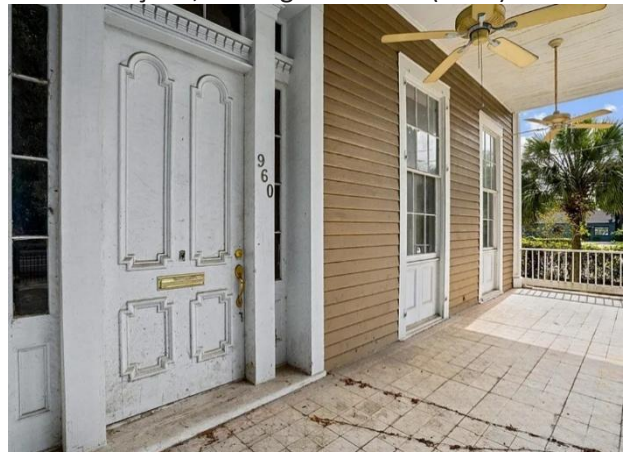
4. Historic entry door, sidelights, and transom (2020)
