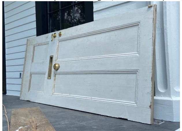
6. Original entry door with new hardware installed
