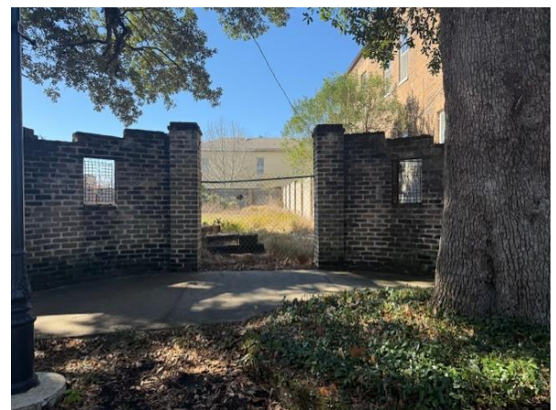
6. Northeast entrance to subject property facing W
