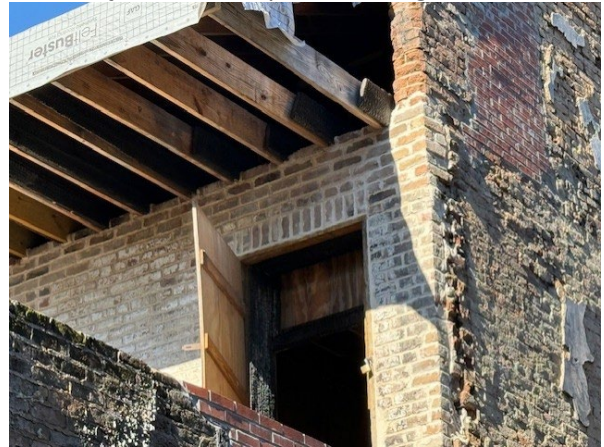
4. Side view; location of addition. Evidence of fire damage.
