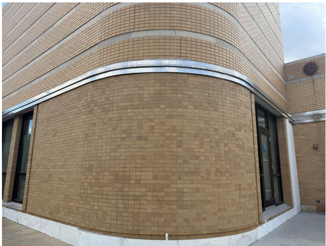
9. View of contrasting and infill brick on north elevation
