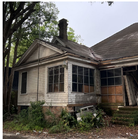
6. Extension on west elevation, location of original porch profile and previous porch enclosure (shingled area)
