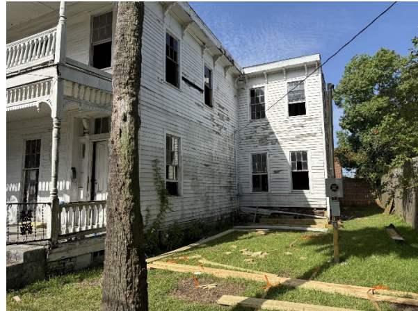
4. View of subject property rear wing, looking west.
