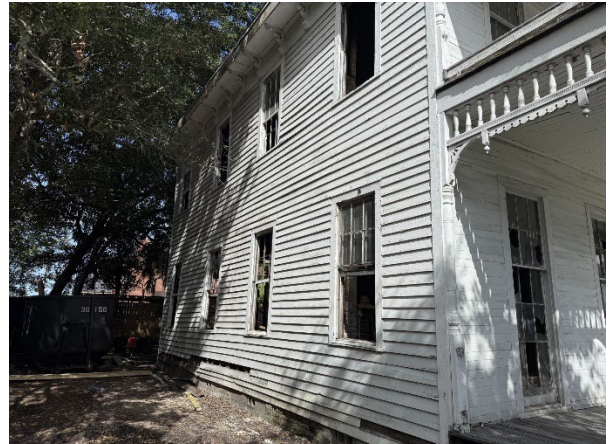
10. View of the south elevation.
