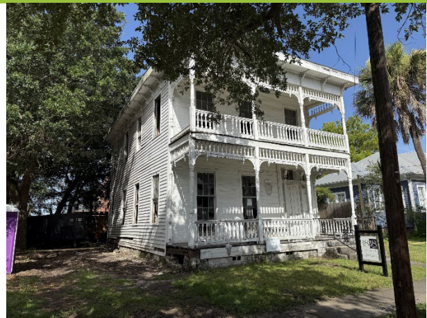
2. View of subject property, looking NW
