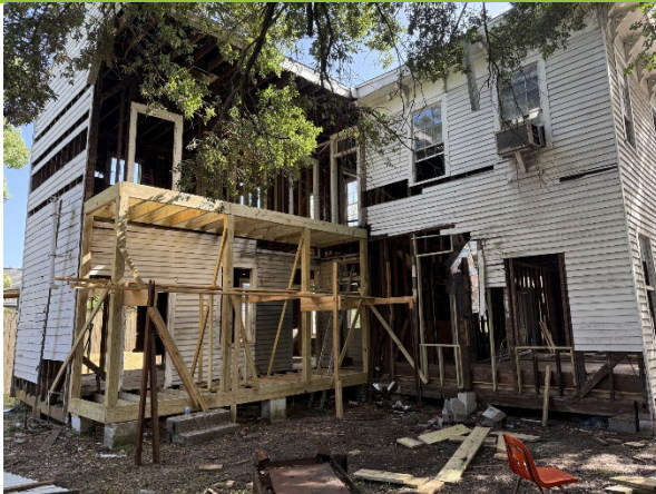
7. View of the west elevation and rear porch.
