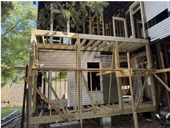
9. View of south elevation of rear porch.
