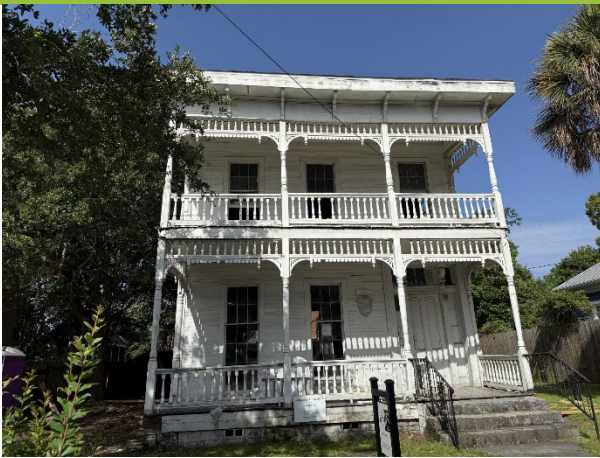
1. View of east façade, looking W.
