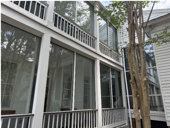
9. Detail of aluminum storefront
