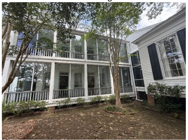
6. View of the west elevation and rear gallery
