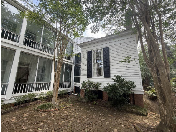
7. View of west elevation and rear gallery
