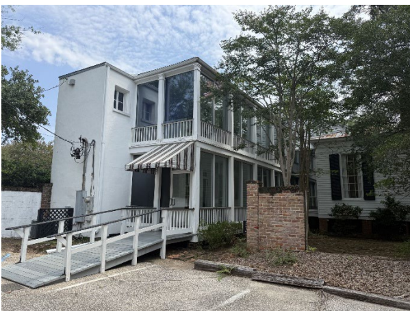
5. View of rear elevation, looking E
