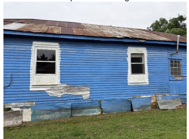
4. West elevation of structure, view of modified window openings.
