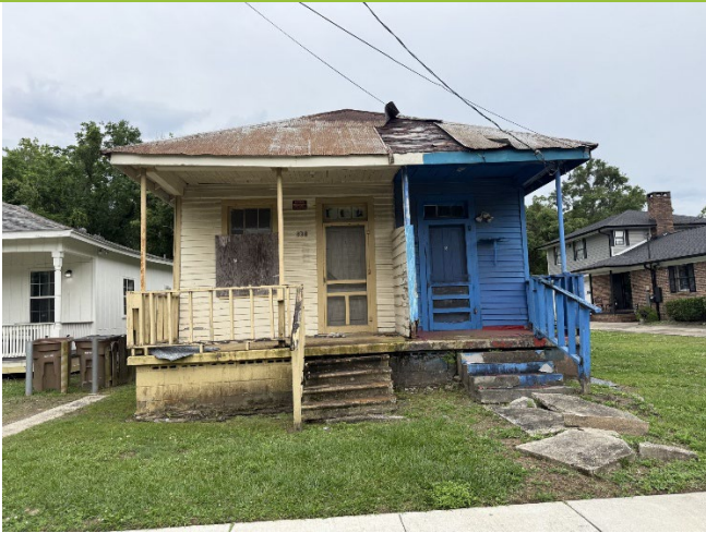
1. North façade, looking S.
