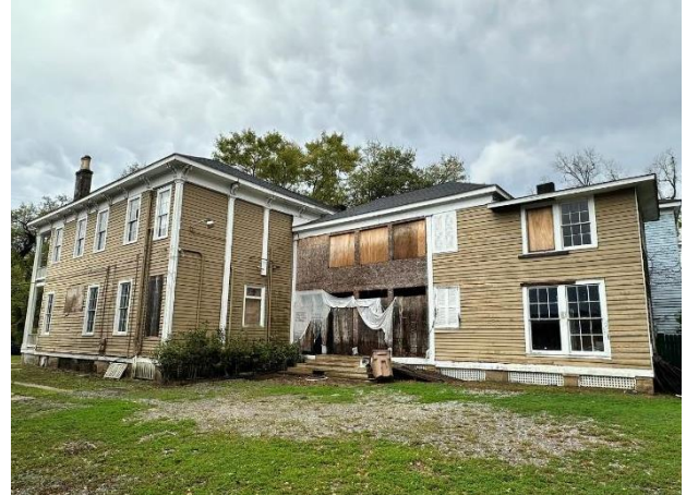
2. East elevation, looking west
