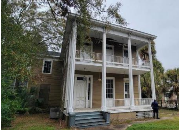
1. Primary (south) elevation, looking north
