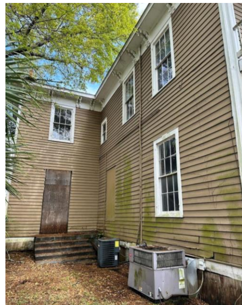
6. West elevation, looking northeast
