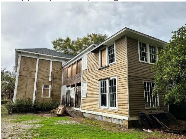
3. North elevation, looking southwest
