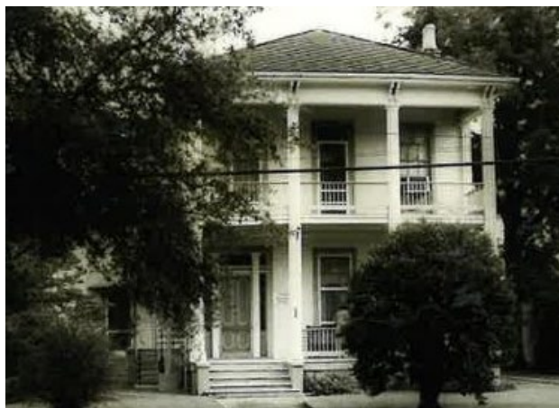
1. Primary (south) façade, looking north (1983)
