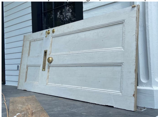
6. Original entry door with new hardware installed
