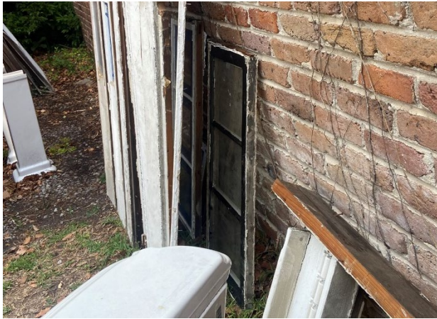
9. Transoms behind door trim pieces
