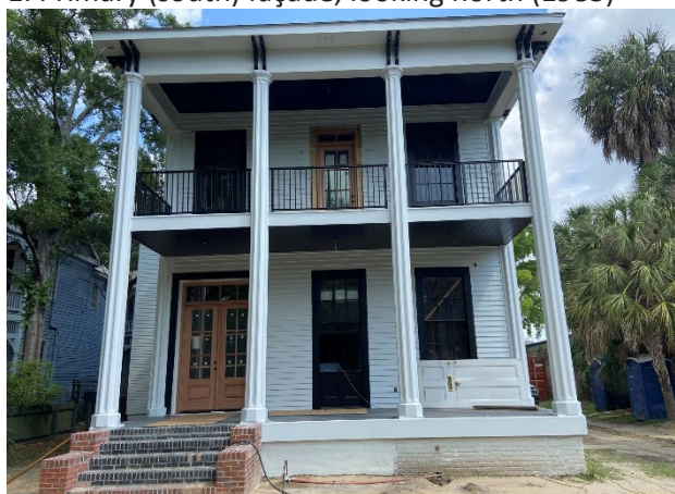
3. Replacement doors (April 2026)
