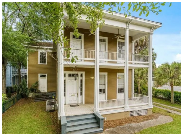
2. South façade, looking northwest (2020)
