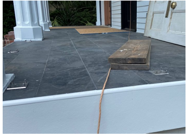
10. New tiles on south porch deck
