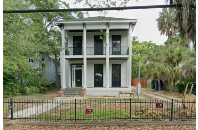
2. South façade, looking north (April 2026)
