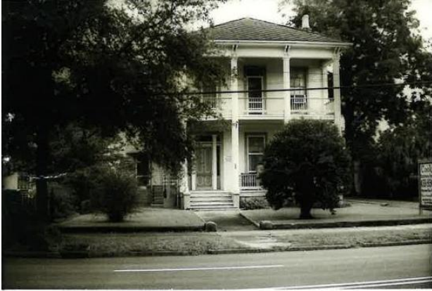
1. Primary (south) façade, looking north (1983)
