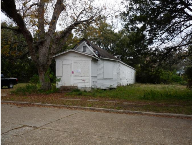
1. View of façade.
