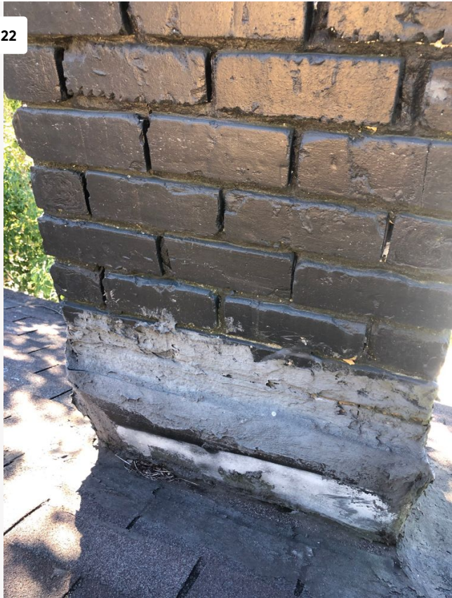
The previous extensive failed repairs show me it is not able to be repaired and properly flashed.
