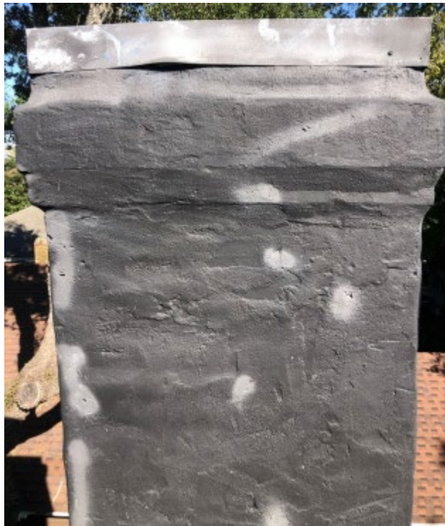
6. Closer view of chimney 1 and the cap that was installed and the concrete that was applied.
