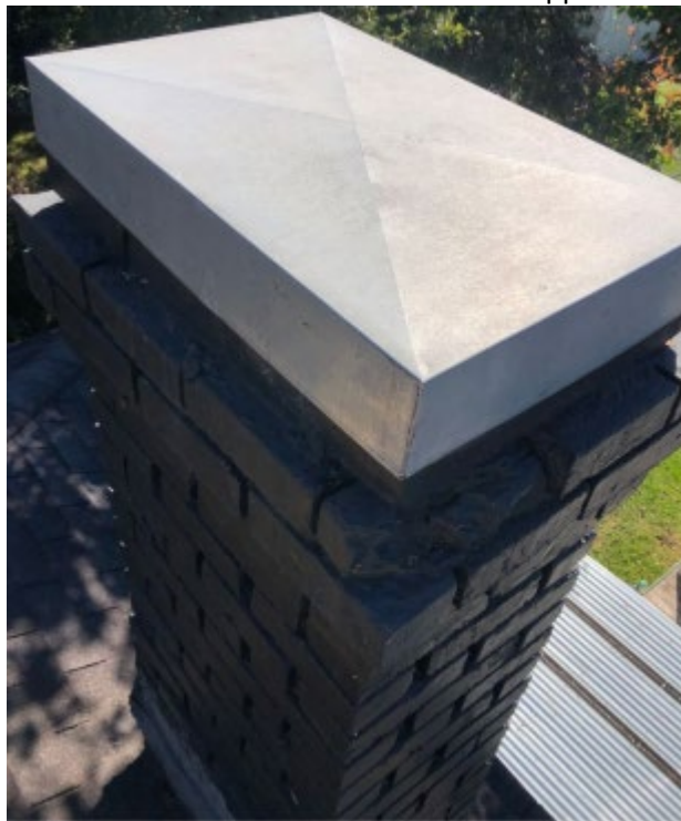
6. Closer view of chimney 1 and the cap that was installed and the concrete that was applied.
