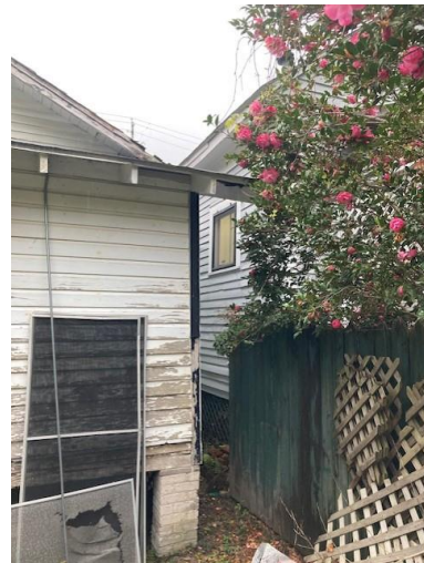
4. View of east elevation, looking SW
