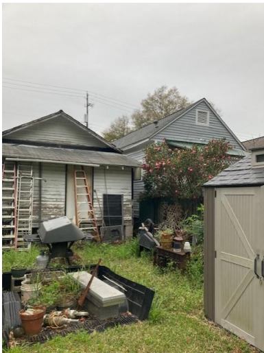
3. View of east and north elevations, looking SW from neighboring property
