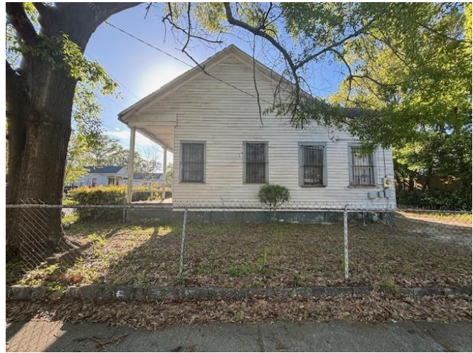
4. View of east elevation, looking west
