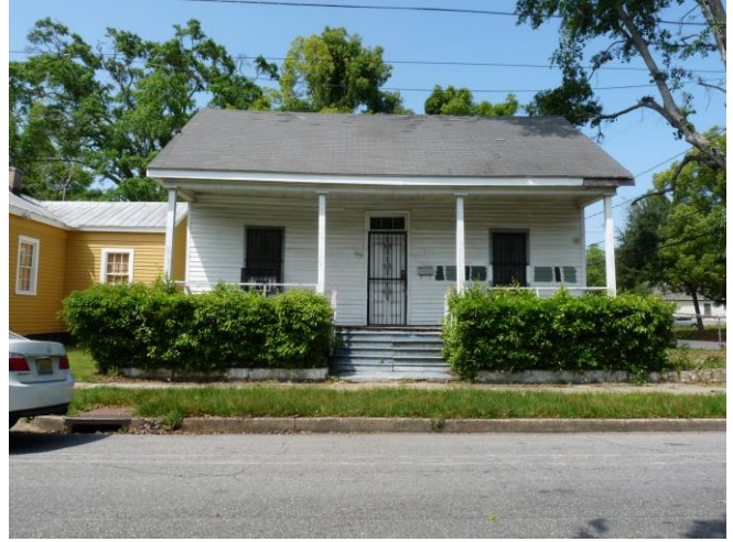
2. View of façade, looking north
