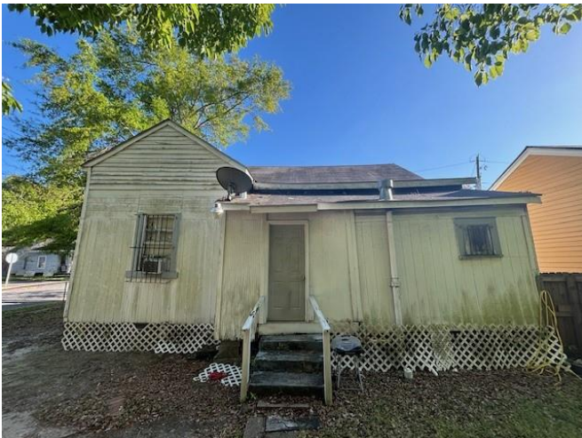
5. View of rear elevation, looking south
