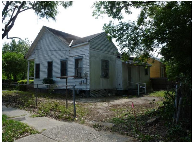
6. View of proposed parking area, looking southwest
