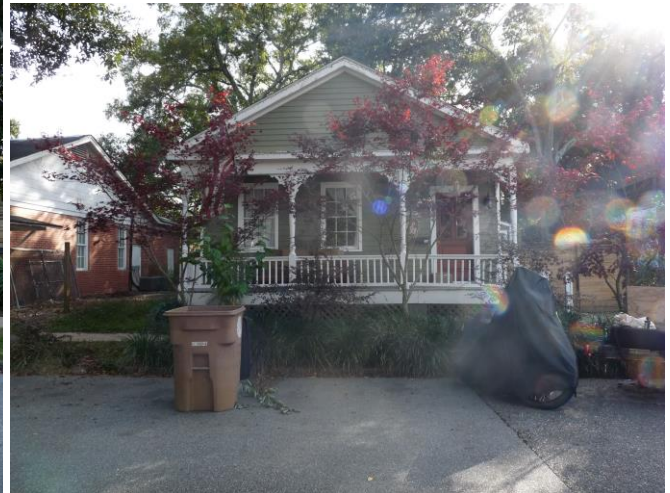
2. North elevation (façade)
