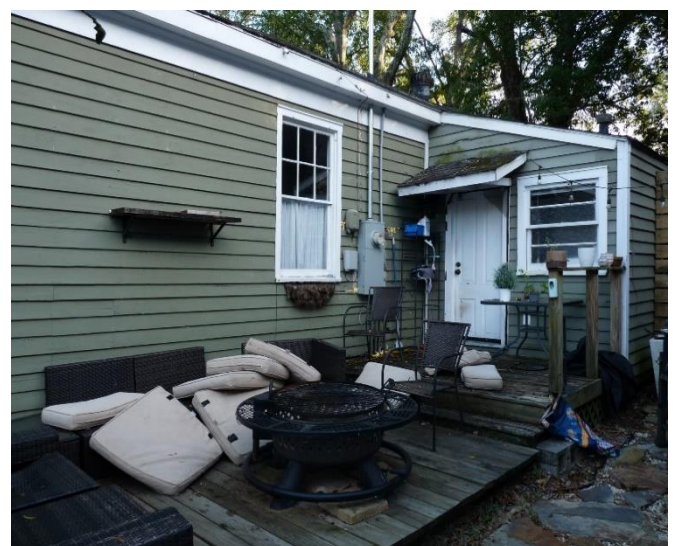
6. Detail view of west elevation, looking southeast
