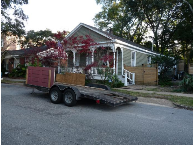
1. North (front) elevation, looking southeast
