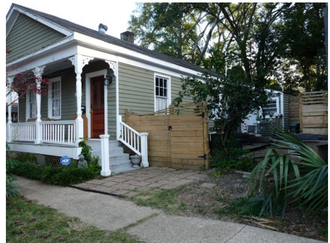
4. West elevation, looking southeast
