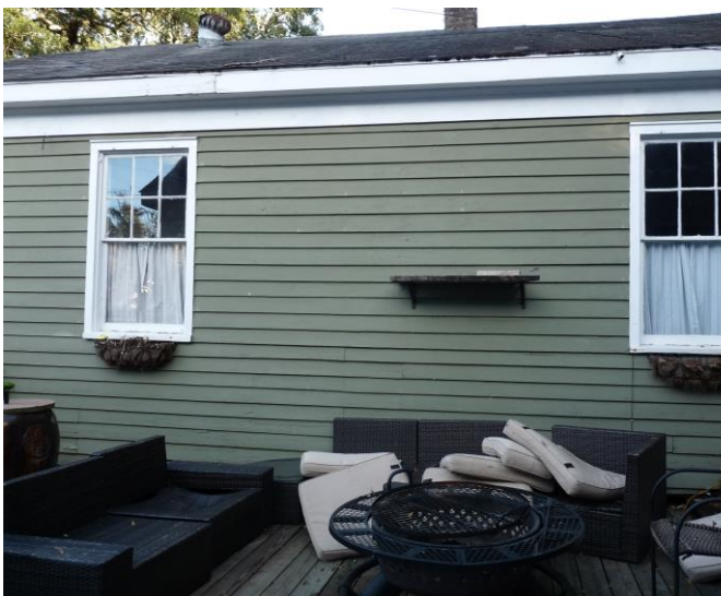
5. Detail view of west elevation
