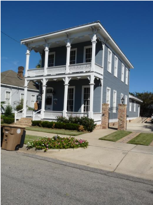
1. View of west façade, looking east by northeast.
