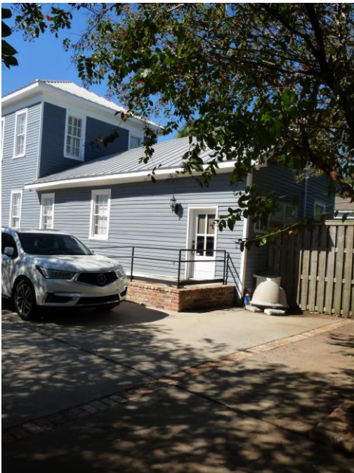
3. View looking north by northwest
