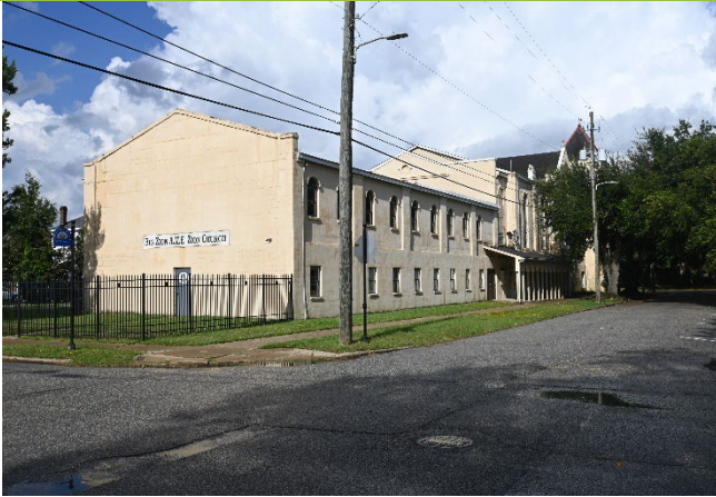
7. View of 115 S Bayou, looking NE from subject property
