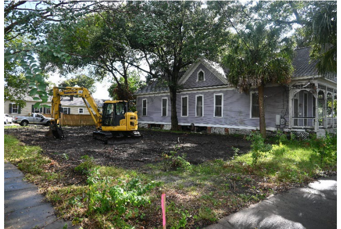
2. View of lot and adjacent structure, looking SW
