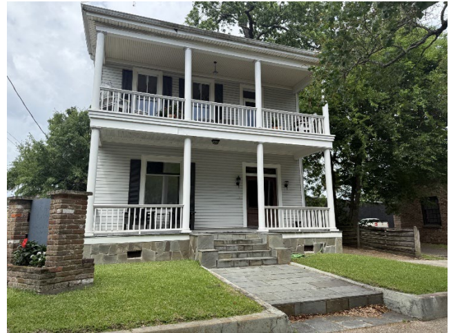
4. View of 7 N Bayou Street (north of subject lot).
