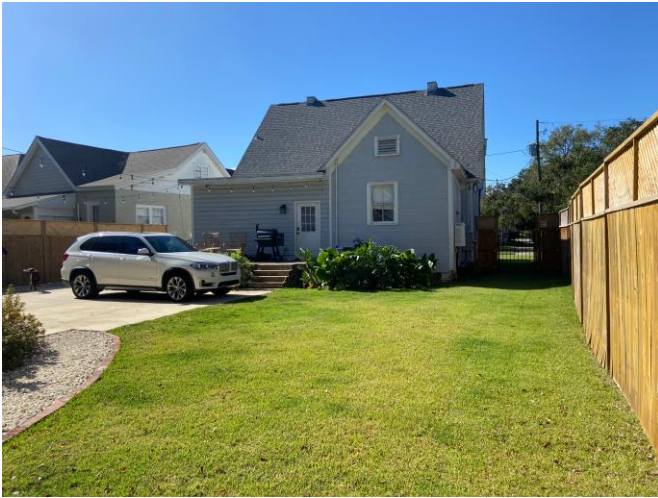
1. View of rear (east) elevation, looking west.
