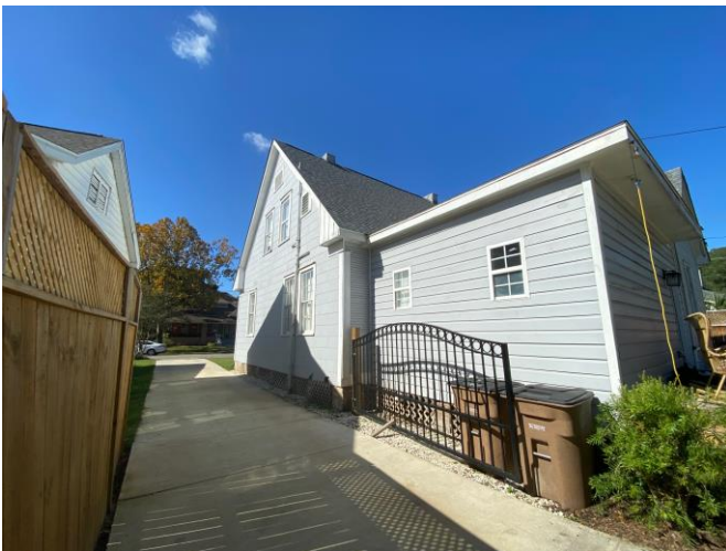
3. View of south elevation, looking northwest
