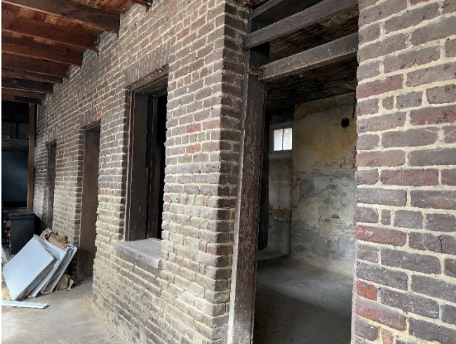
1. View west-northwest along south wall of 1 st floor porch, rear wing
