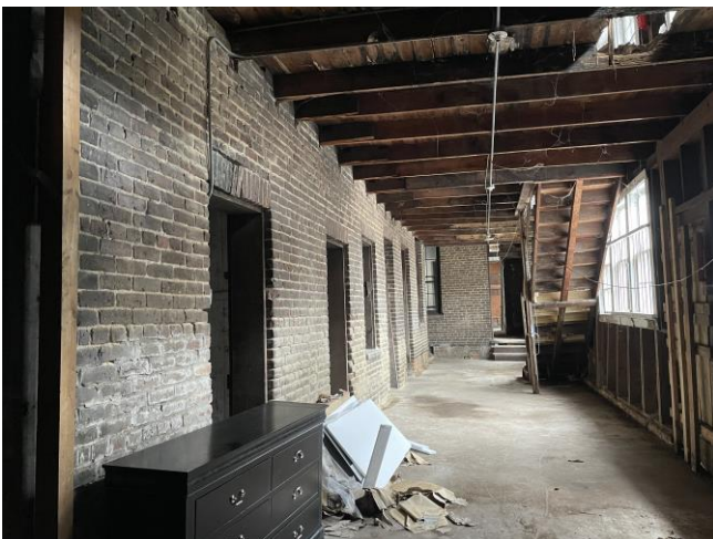
5. View east along south wall, 1 st floor porch, rear wing
