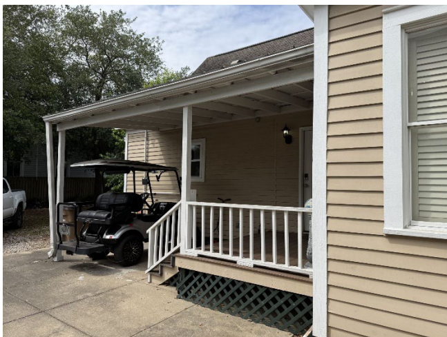
5. Shed roof projection on east elevation, looking SW.
