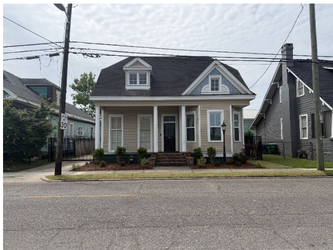
1. View of North façade looking S.
